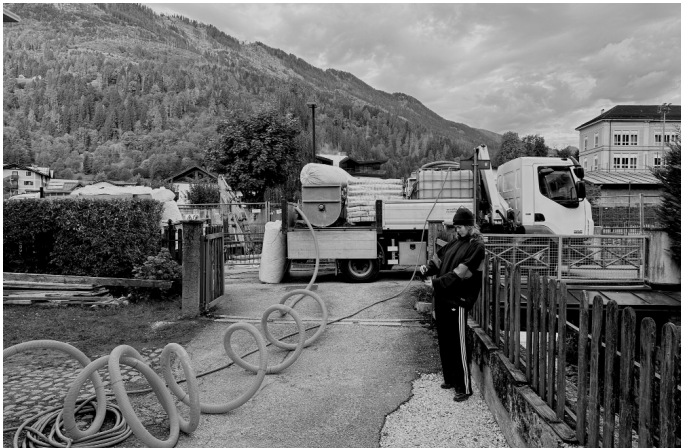
View of the driveway, a day on the worksite
